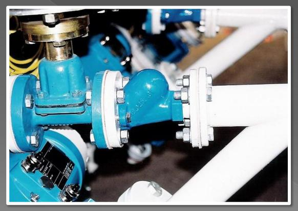
Mechanical fail safe Non-Return Valve for protection against delivery line run-back during process shutdown or emergency stoppage.
