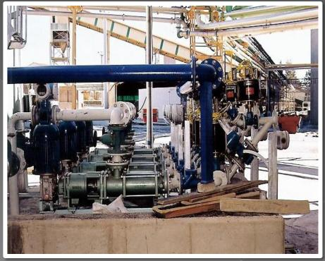
C-15 with the an enclosed flocculant loading and storage facility located above the sequence tanks.
