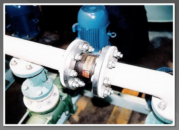
Dangerous pressures can occur within delivery lines. Rubber Explosion Safety Couplings protect against catastrophic failure and dangerous pipe bursts in the event of unexpected damage or blockage of remote delivery piping.
