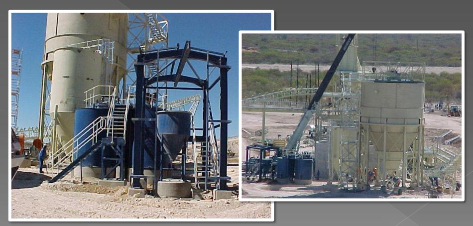
C-15 with the flocculant loading and storage facility located next to the sequence tanks.
