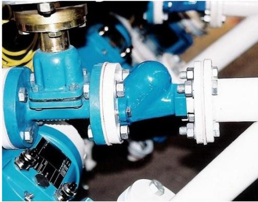
**Non-Return Valve-** mechanical fail safe non-return valve for protection against delivery line run-back during process shutdown or emergency stoppage.
