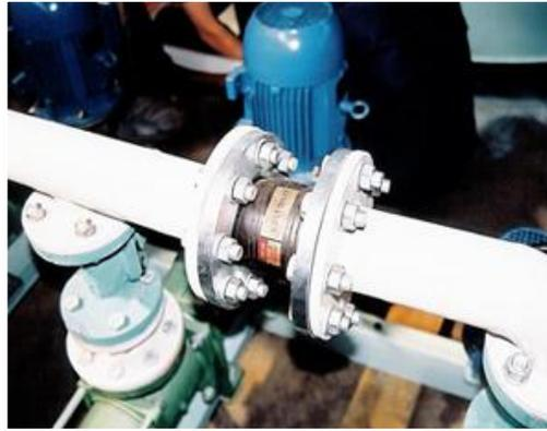
**Explosion Coupling-** Dangerous pressures can occur within delivery lines. Rubber explosion safety couplings protect against catastrophic failure and dangerous pipe bursts in the event of unexpected damage or blockage of remote delivery piping.
